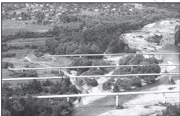
Fig. 8.17: Pipelines transporting natural gas in Ukraine
